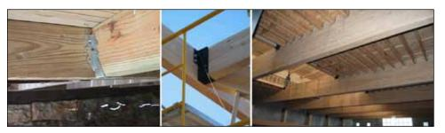
Figure 8-28. Typical joist hanger connectors.
