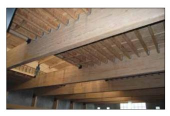
Figure 11–1. Wood-based composites used in the new Centennial Research Facility at the Forest Products Laboratory. Glulam timbers support composite I-joists and plywood sheathing. (Photo by Steve Schmieding, Forest Products Laboratory.)
