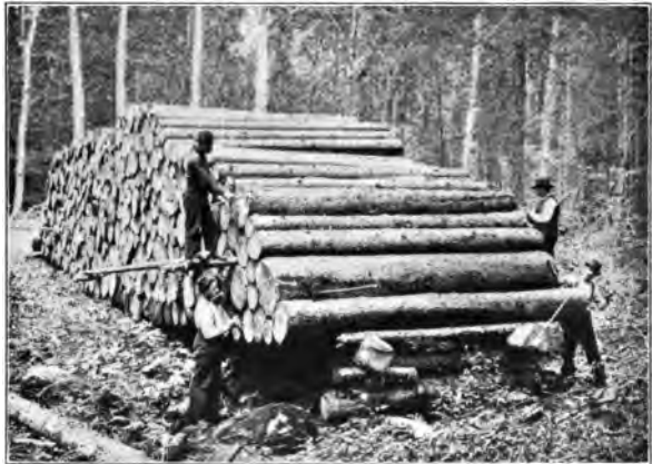
Fig. 9. "Scaling" Logs on the Skids.
