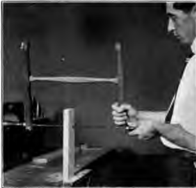
Fig. 95. Using a Turning-Saw.
