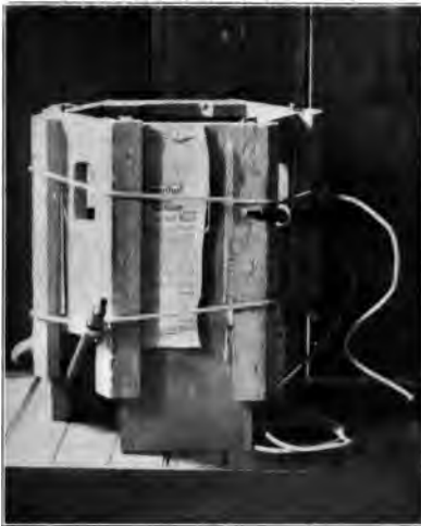
Fig. 257. One Method of Gluing up a Six-Sided Taboret.
