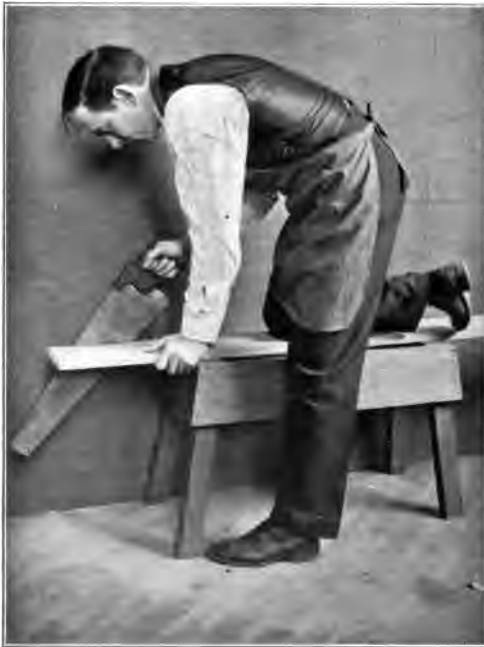
Fig. 88. Rip-Sawing on a Horse.
