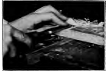
Fig. 71. Chiseling Out a Dado (Second Step).
