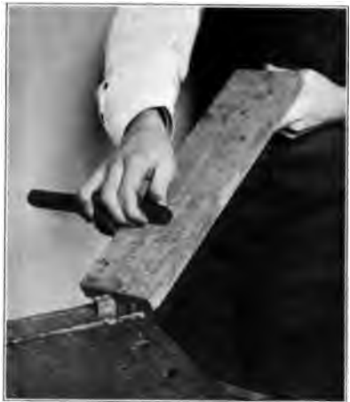
Fig. 214. Using the Marking-Gage.
