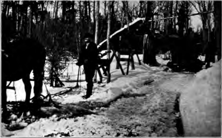
Fig. 10. Making an Ice Road by Flooding.
