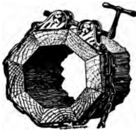
Fig. 259. Column-Clamp.
