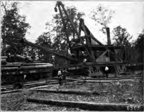
Fig. 27. Steam Skidder at Work. Grant County, Arkansas.
