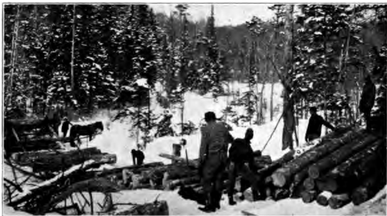
Fig. 12. Loading a Sled from a Skidway.
