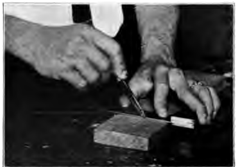
Fig. 204. Scribing with Knife by Try-Square.
