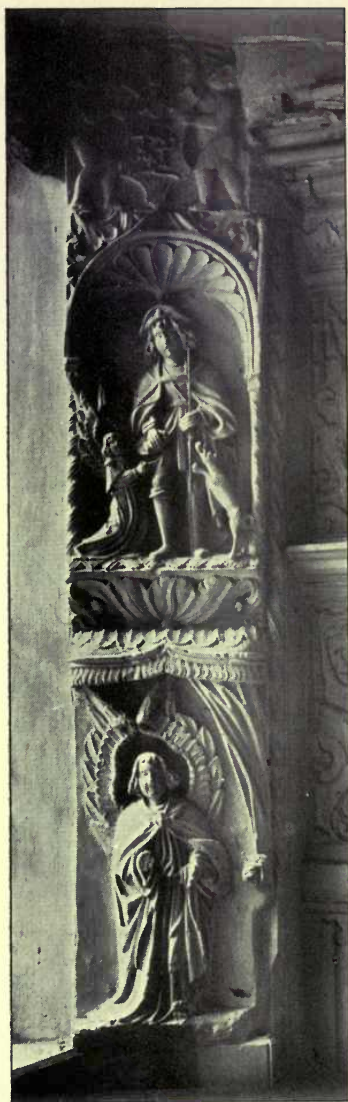
Panels on the South side of the Window.
